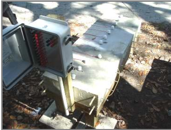
Figure 8 - Installed yard slab with connection box.
